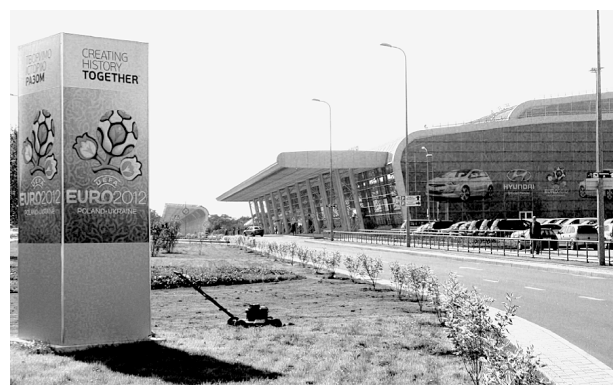
Fig. 21. New airport terminal. (© Bohdan Posatskyy, 2012)
