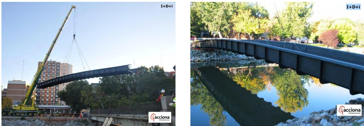
Fig. 1. (a) Installation of the FRP girder; (b) View of the Almuñecar footbridge (Courtesy of Acciona Infr.)
