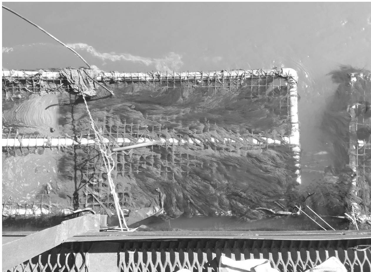
Fig. 1. Rafts with fibrous carrier of the “VIYA” type installed at the sludge collector of the “Zaporizhstal” PJSC plant
