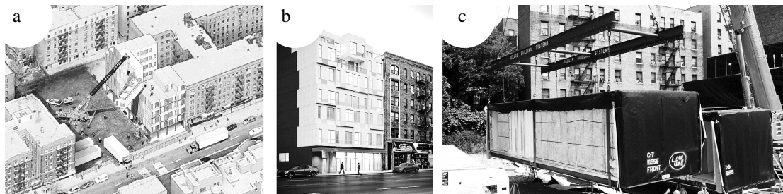
Fig. 2. Method of mounting modules from the adjacent area using a crane (a); appearance of the external facade and volume (b); unloading of the assembled modules at the construction site in New York, USA (C) (The Stack Modular Housing in Manhattan / Gluck + [Electronic resource] // ArchDaily. – 2020. – Resource access mode: https://www.archdaily.com/943491/the-stack-modular-housing-in-manhattan-gluck-plus?ad_source=search&ad_medium=search_result_all )
