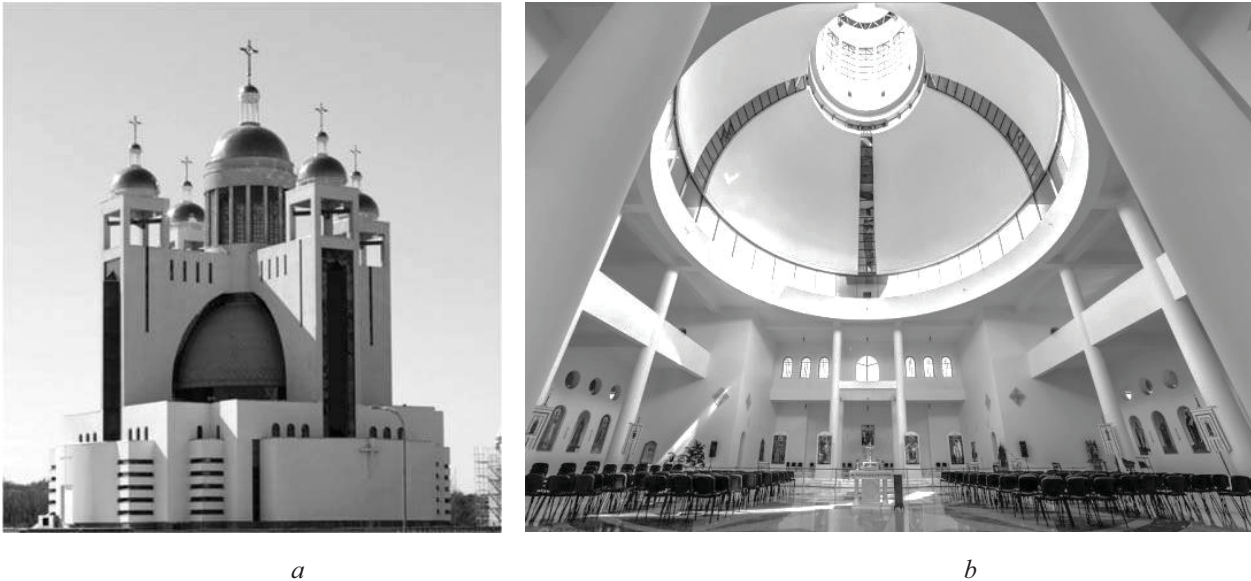
Fig. 3. Facade (a) and interior (b) of the Patriarchal Cathedral of the Resurrection in Kyiv [III]
